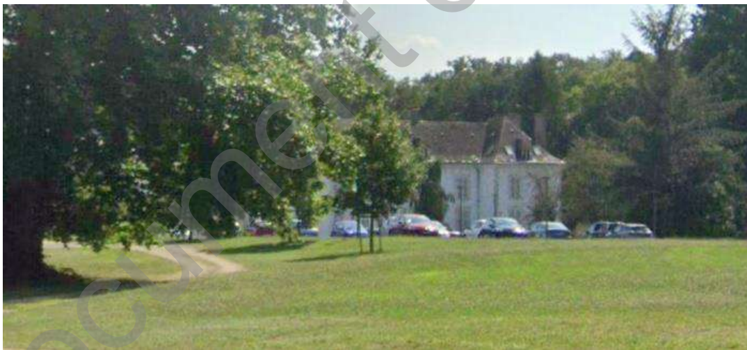
Photo 55. Château de Villecante (Google Street View)
